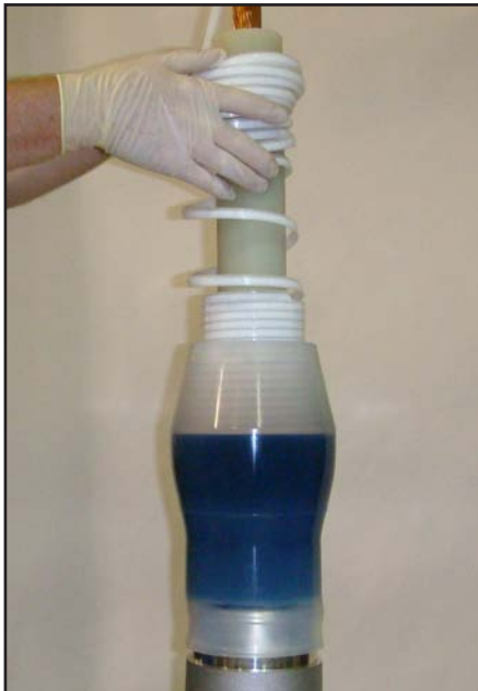
▲ Mechanical shrink stress cone
