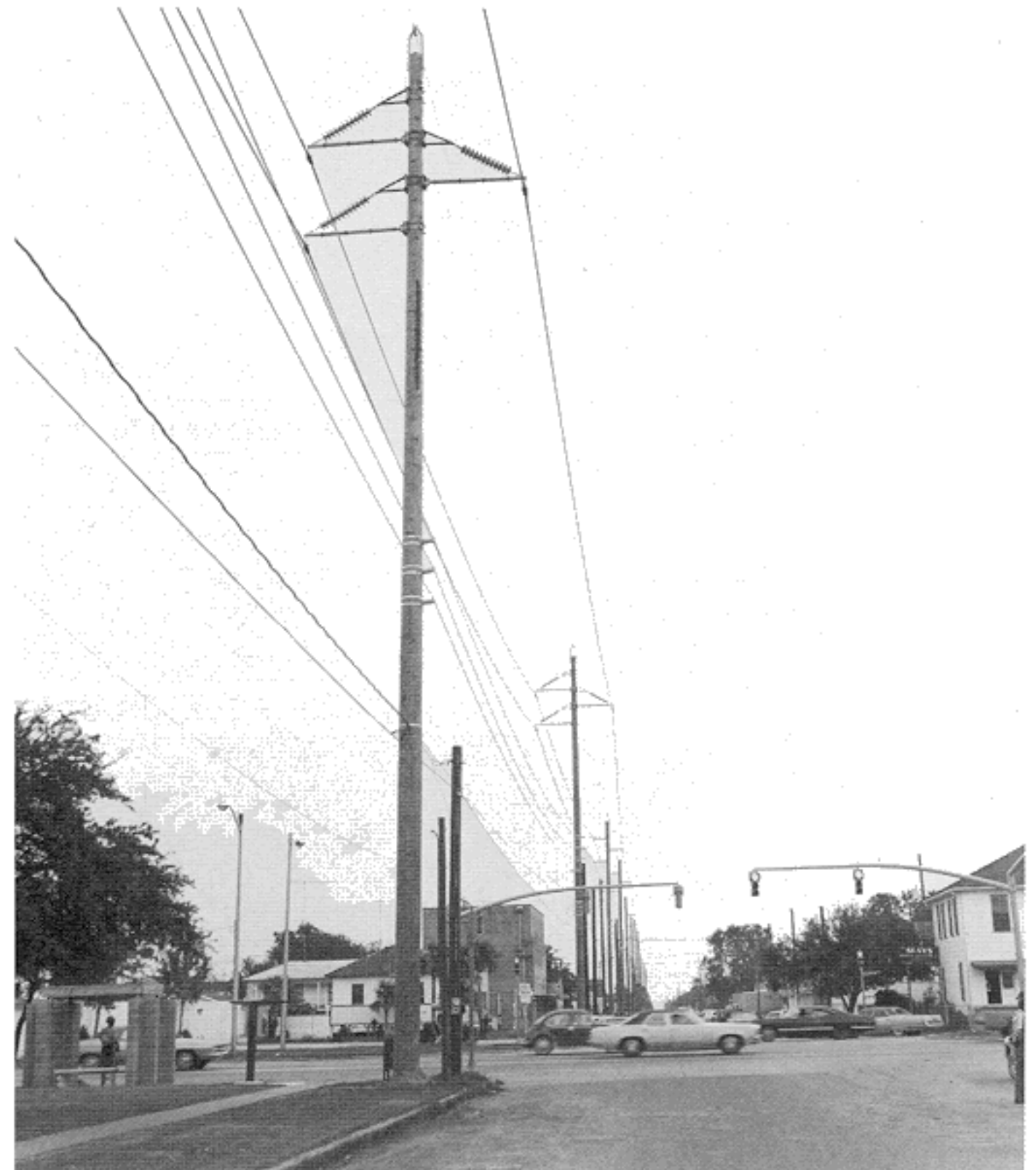
Overinsulated 138 kV Horizontal Vee line through a seacoast city illustrates the versatility of the design. The Horizontal Vee assemblies were mounted in a delta configuration on wood poles with tie-bands to prolong the life of the treated poles.
