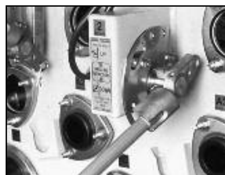
▲ Fault interrupter operating handle.
