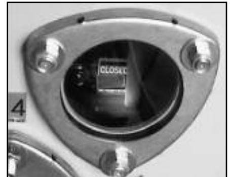
Position indicators (right) provide contact position indication through viewing windows. ▶
