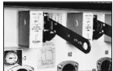
▲ Single phase interrupter operating handles.
