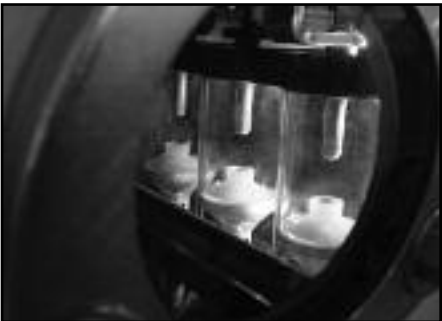
▲ Load break switch visible break.
