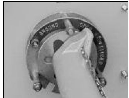
▲ Load break multi-position switch operator.
