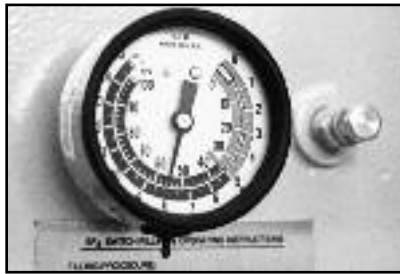
▲ Pressure gauge and fill valve
