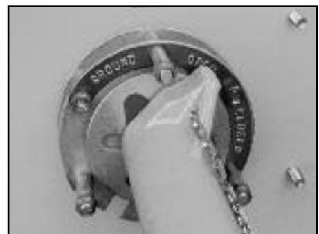
▲ Load break multi-position switch operator.
