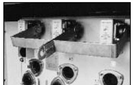
▲ Three phase interrupter operating handle.
