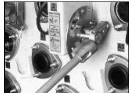
▲ Fault interrupter operating handle.
