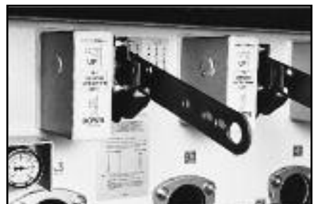
▲ Single phase interrupter operating handles.
