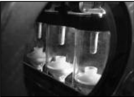
▲ Three phase visible position of contacts.
