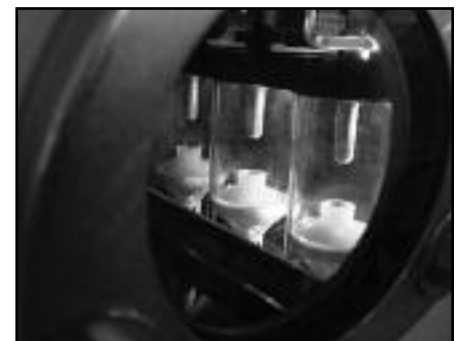
▲ Load break switch visible break.
