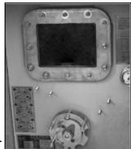
▲ Load break multi-position switch operator.
