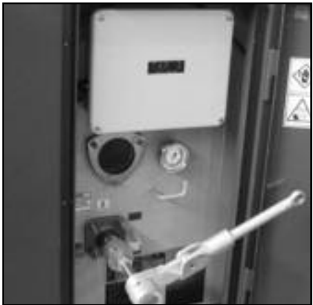
▲ All load break switch operators are located on the side of the switch.
