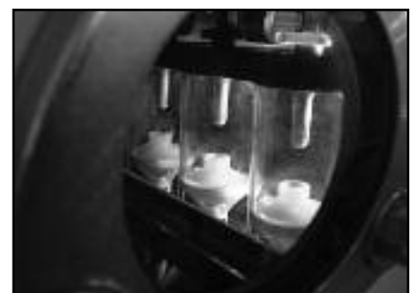
▲ Load break switch visible break.
