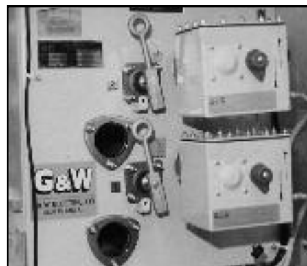
▲ Cock-and-trip switch with manual operating handle.
