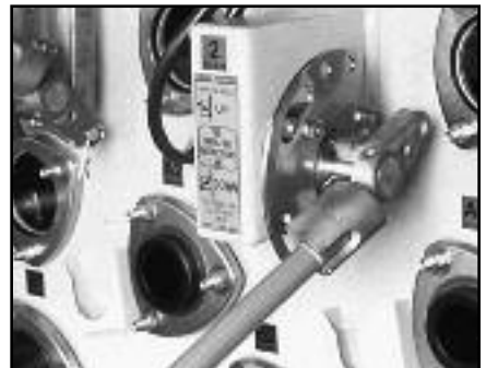
▲ Fault interrupter operating handle.
