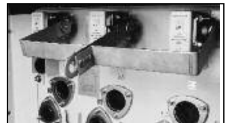
▲ Three phase interrupter operating handle.
