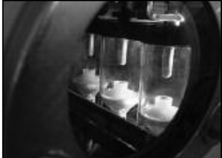
▲ Load break switch visible break.
