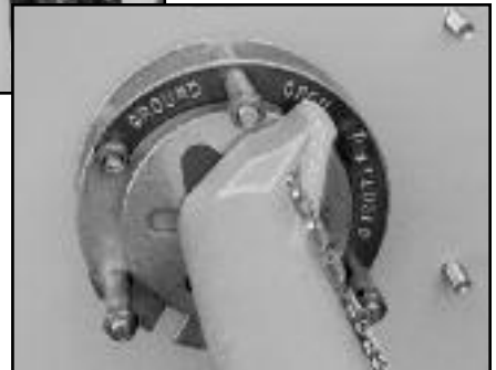
▲ Load break multi-position switch operator.
