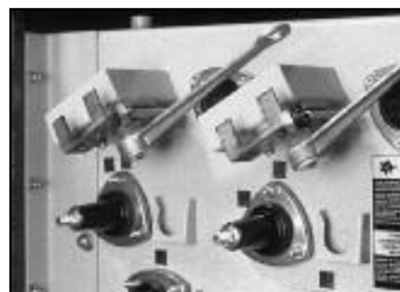
▲ Hookstick operable load break handle.
