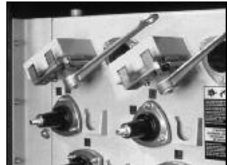
▲ Hookstick operable load break handle.
