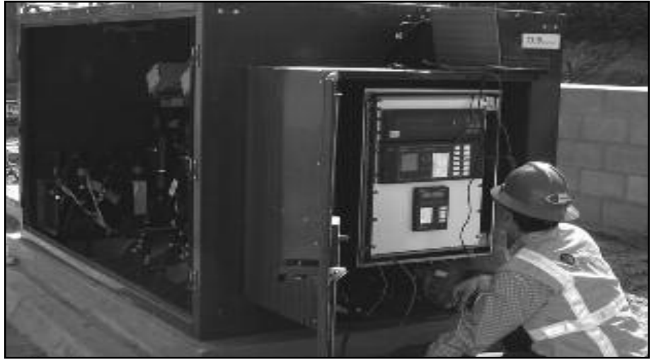
▲ Padmount switch with SEL controls.
