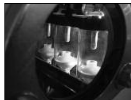
▲ Load break switch visible break.
