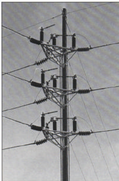
69 kV "3D"-600A switch on wood pole. ▼
