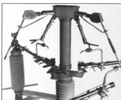
3. Bypass disengaged, circuit interrupted. ▲
