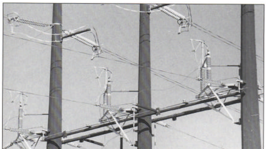
Unique Horizontal Phase-next-to-Phase base and frame construction. 2 way switch shown, also available in 3 way configuration. ▲
