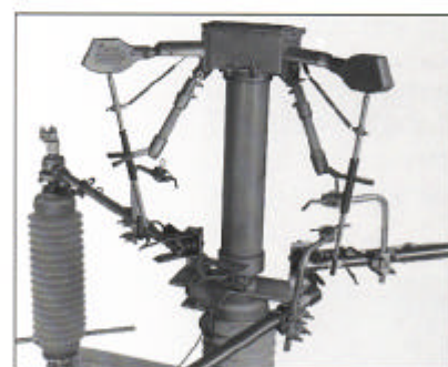
2. Switch starts opening, Bypass engaged. ▲
