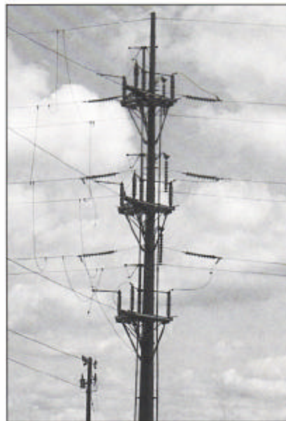
1200 Ampere, 138 kV "3D" automatic motor-operated switch on steel pole. ▼
