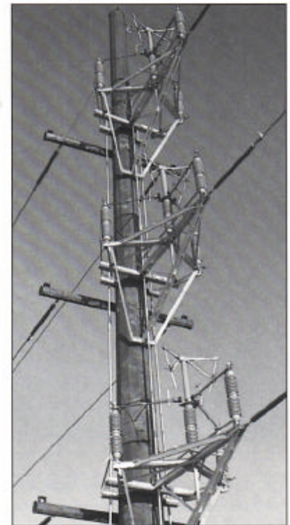
1200 Ampere, 161 kV "3D" switch on corten pole. ▼
