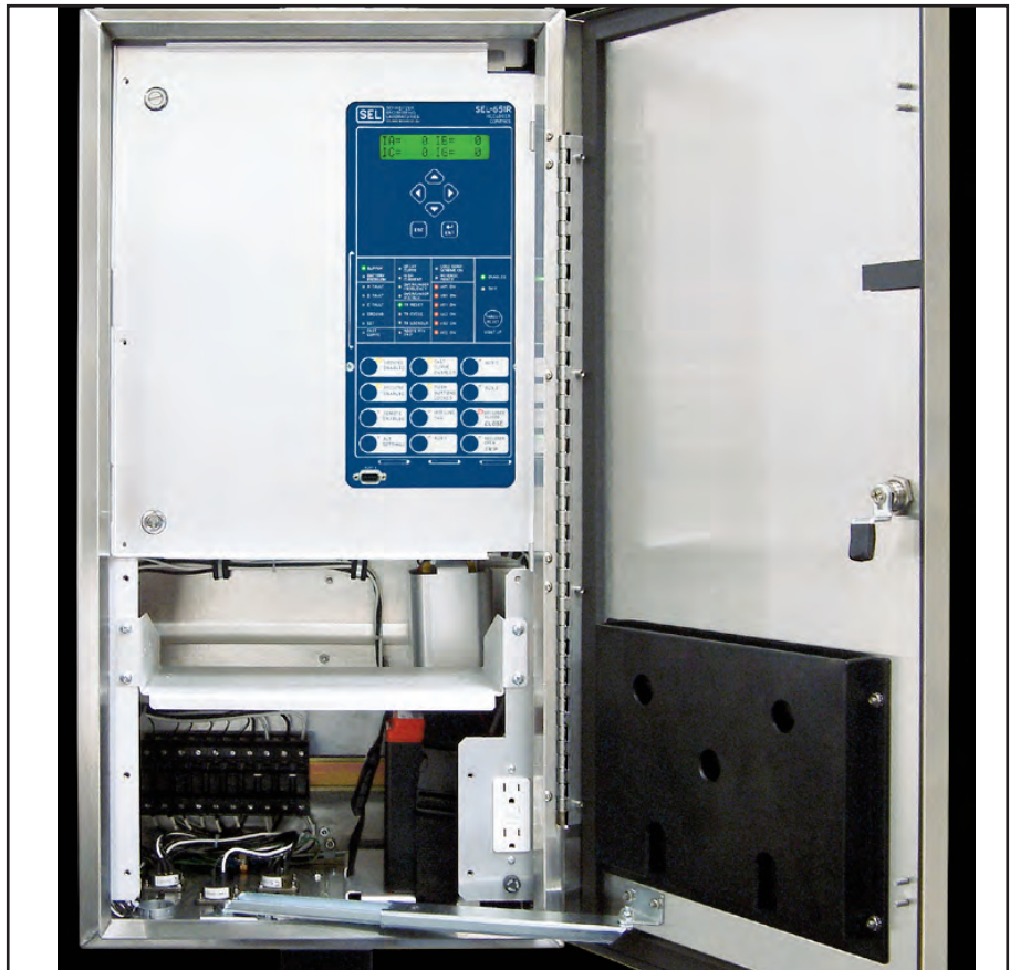
▲ Schweitzer SEL-651R front access control (above) for conventional recloser applications. Front/back access control cabinets are available.
